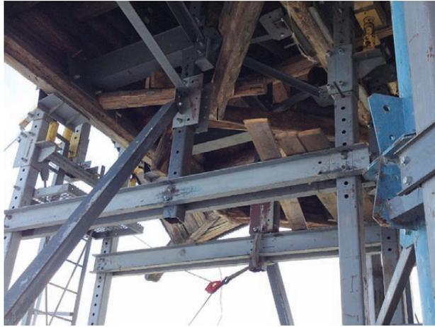
*The lifting structures supporting the upper suspended part of the church were re-mounted*
