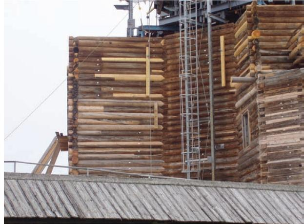
*Tightening of annexes walls with cord strainers and wooden binding posts*
