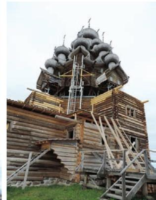
*Assembly of the 5<sup>th</sup> restoration tier on the Pogost site*
