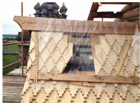
*Making roof eaves and covering for the “barrel” roof of the altar dome*
